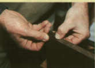
Photo 9. Fitting the hinge in the mortise on the door edge.
