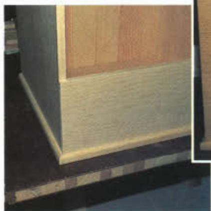
Photo 7 The simple addition of a base shoe molding helps make the piece more pleasing to the eye.
