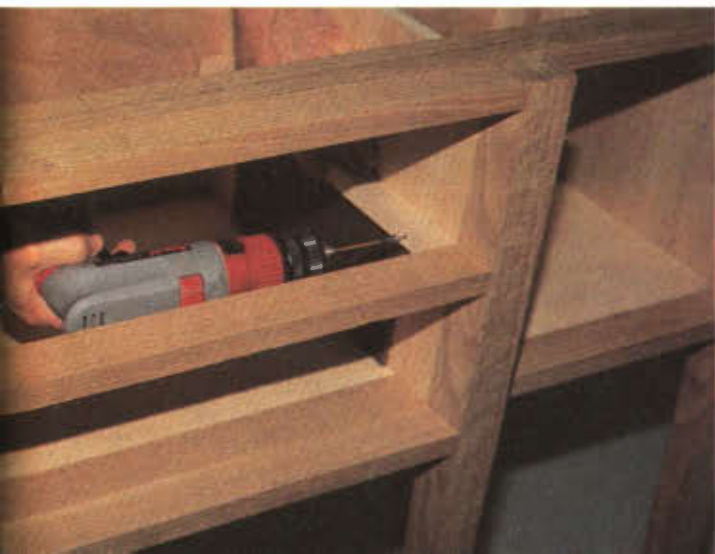
Photo 10 The upper drawer requires cleats for drawer slides. Simply screw a piece on that's flush with the top edge of the middle rail. I used a spacer to position the rail while it was screwed in place. The bottom drawer rides on the case bottom. Since the partitions are set flush to the leg and square to the front, the drawers are captured between them. Sizing the drawers is just a matter of deducting ¼" from the overall drawer opening size to allow for side to side and top to bottom clearance.
