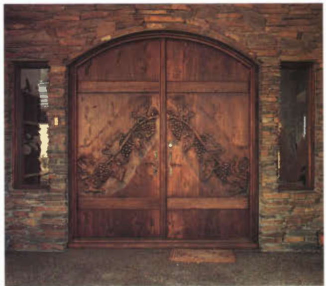
Photo 1. Another double door entryway by the author shows a book matched design using plank construction technique.
