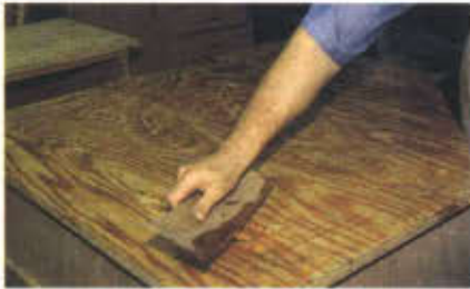
22. Contact cement may also be spread using a notched spreader. This is a shop-made version of scrap laminate.
