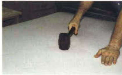
23. A rubber mallet does fine to start the contact, but it's difficult to make sure you have covered the entire surface. Follow up with a roller.
