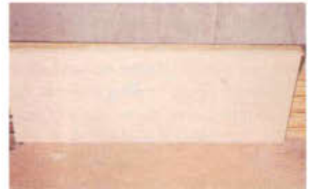
Photo 9. A decorative bead can be used on the edge of the liner to provide a more attractive finish.
