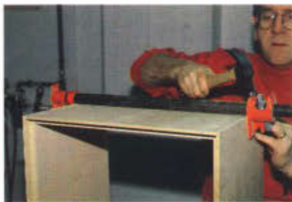
Photo 6 Cabinets are assembled with glue and nails. A clamp pulls the parts together while fastening.
