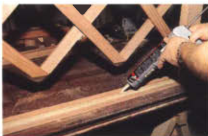
Photo 2 A dab of paneling adhesive is used at every location where the slats enter the groove in the frame.
