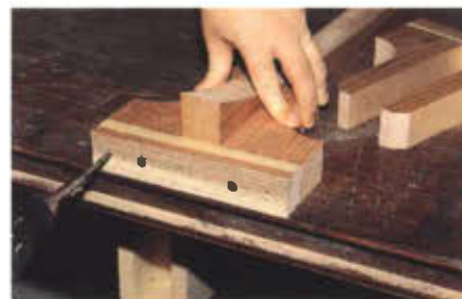
Photo 3 The U-shaped brackets are glued and screwed together using a frame stile to determine the proper spacing.
