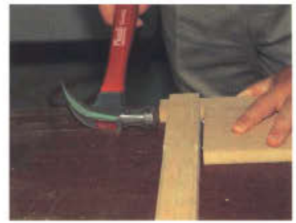
Photo 9 The doweling centers (the metal pieces between the apron and leg) are placed in the dowel pockets in the apron. By lightly tapping the leg against the centers, a visible indentation is made to guide the drill for the opposing dowel pockets.
