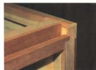
Photo 10 The redwood cap and trim must be notched to fit.
