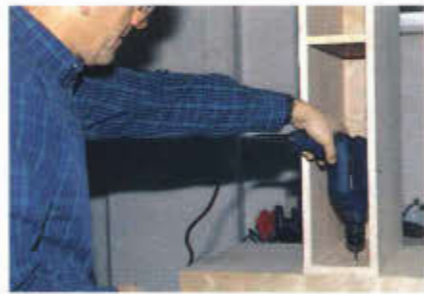
Photo 8 The saw table platform cabinet is screwed to the back of the router cabinet.
