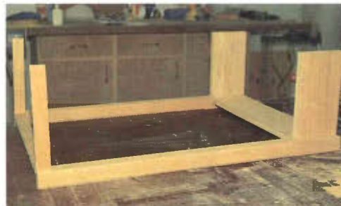
Photo 12 The end aprons and kick pieces are doweled first to one frame, lying flat.
