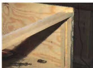
Photo 9 The sliding door track is formed by attaching strips.
