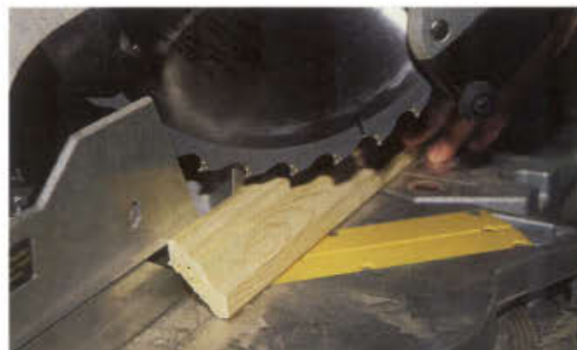
Photo 1 Place the crown molding between the fence and table at a 45° angle in the same position as it will be mounted. Set the saw to make a 45° cut. By doing this, a compound cut is made.
