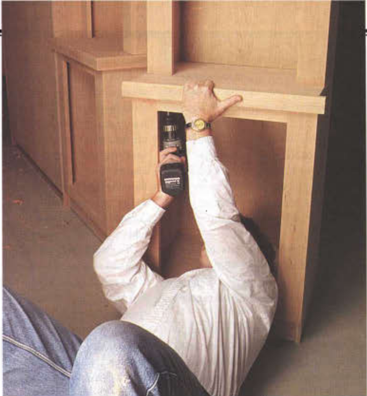
The assembled upper cabinet is secured to the lower cabinet by screwing up through the mounting strips into the counter tops. Make sure you use the right length screw!
