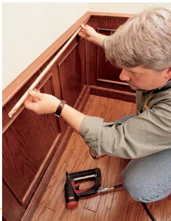
The last step is fitting and tacking the cove moulding strips in place. Note on the leading edge of the moulding. The 45-degree cut is half of a scarf joint.
