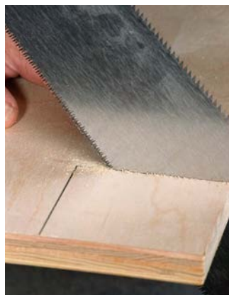
Before assembly, handsaw 3" x \frac{3}{4} " notches in the sides at the bottom corners to make the toe kick space.
