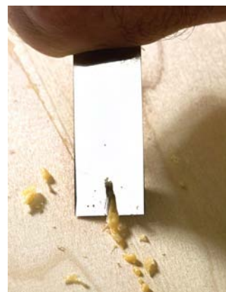
When the glue is soft but no longer a liquid, peel it away with a chisel. Make sure your chisel is sharp.
