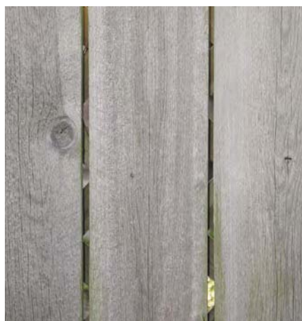
The combination of sunlight and rain causes wood to turn silvery gray. If you like the gray color, and you aren't having other problems, you can leave the wood unprotected. The grayed surface is very effective at blocking further degradation below. UV light erodes wood at only about 1/4" per century.
