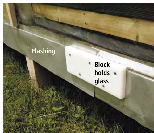
The bottom of the wall windows rests on a 1/4" ledge in the framing. Aluminum flashing keeps water out while the glass is held in place by a block, in this case scrap Corian left over from a countertop installation.
