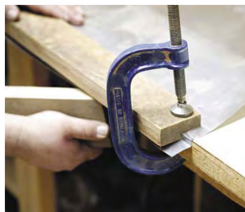
Bending the aluminum flashing used in the 1/4" ledge on which the window wall glass will rest. Step one was to make a right angle in the flashing. Here, the final bend is facilitated by a board with a 1/4" rabbet sawn in it and clamped to the bench.
