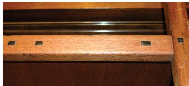
There's a reason for that. The wider pegs at the outer ends of the shelf rail conceal slots for screws. Under the smaller pegs in the middle, the screws are in holes.
