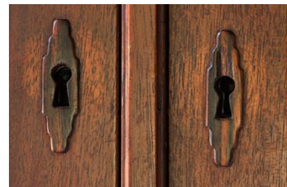
Handmade hardware. Certainly, commercially available hardware would have been cheaper and simpler, but the Greens often designed theirs instead, as in these escutcheons.
