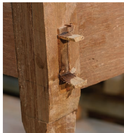
I meant to do that. The story of this joint stretches back nearly a year to the beginning of this series. The first thing I did was undercut this leg. A hasty repair was a recognition that I was in over my head with this project. As bad as this joint looks, the wedges are actually not repairs.
