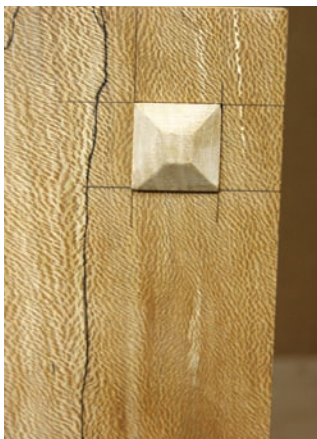
One is good. Here is the joint, assembled on the first try.
