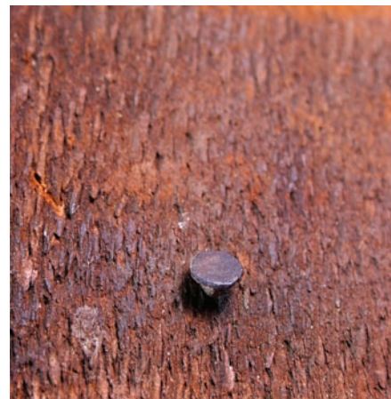
Wrong nail. Wire nails, which have a round shank and a round head, were invented in the 19th century and have no place on an early piece such as this—unless they were added to repair a piece.
