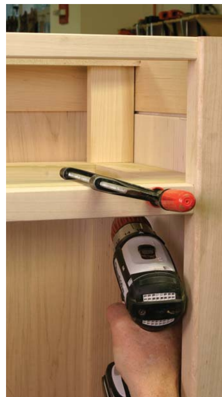
Simple fix. A pocket screw at each end attaches the drawer frame to the inside of the back legs.
