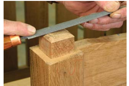
After the fit. Mark the intersection of the arm and the tenon with a pencil line and round the end of the tenon down to the edge. Stop just outside the line to maintain the fit between the two parts.
