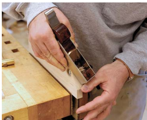
Shoot the stick. Plane the mitered end of the stick in the miter jack.
