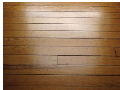
Polyurethane. Among consumer finishes, oil-based polyurethane, shown here on a pine floor, wears best of all finishes.
