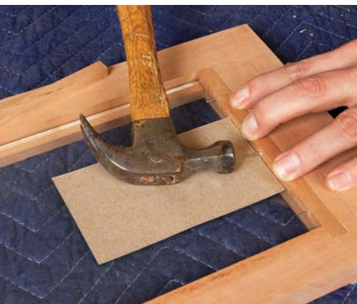
Install the glass. A bead of silicone and wood strips secure the glass in place. Use cardboard to protect the glass as you tap the brads home.
