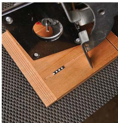
Two passes. After routing a narrow groove between the field and the crossbanding on the top, reset the fence for a second pass the exact thickness of the banding for a snug fit.
