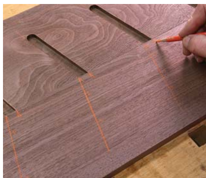
Exacting layout. The best way to mark for the opposing-angled dados for the center divider is directly off the cabinet side.
