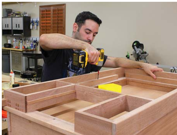
Second time around. Another set of cleats help hold the base firmly to the deck and case.
