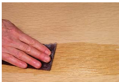
Scotch-Brite scrub. The spill was still distinct after the some light sanding, so I gave it a light scrub with a Scotch-Brite pad and more soap finish. Ideally, I would have done this to the entire surface to ensure an even coloring.
