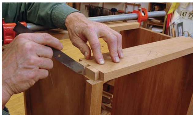
Tails on top. After adjusting the length of the top rails, cut the dovetails. With the rail in place, mark the sockets.
