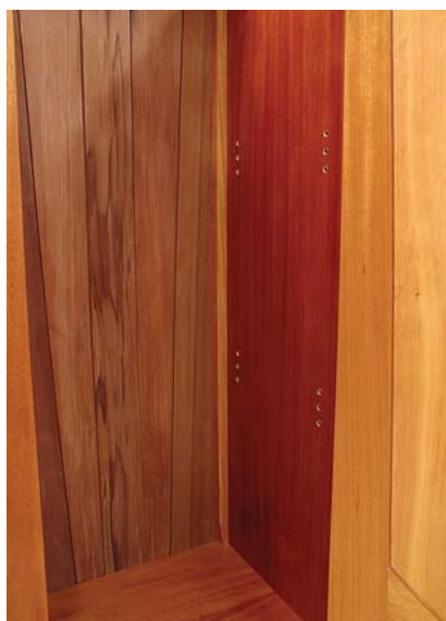
Tapered, too. To continue the overall design, the outer slats of the back are also tapered.
