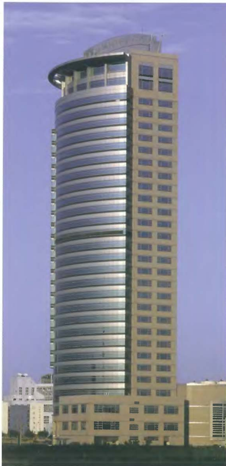
138 Bank of China Regional Headquarters
