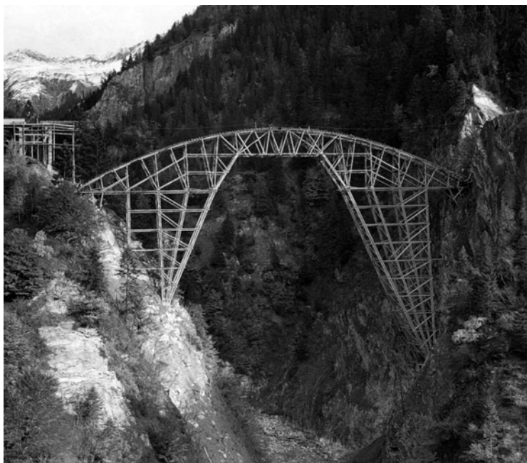
FIG 8. Centring for the Salginatobel Bridge, Switzerland
