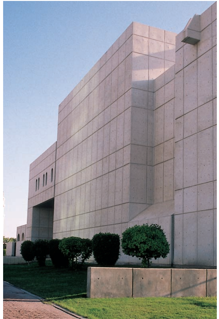
Right The Cultural Foundation, National Library and Cultural Centre: details of the white fair-faced concrete façade. The rendering of the exterior is mastered by a line of discreet and impressive design that has not been matched in style and form
