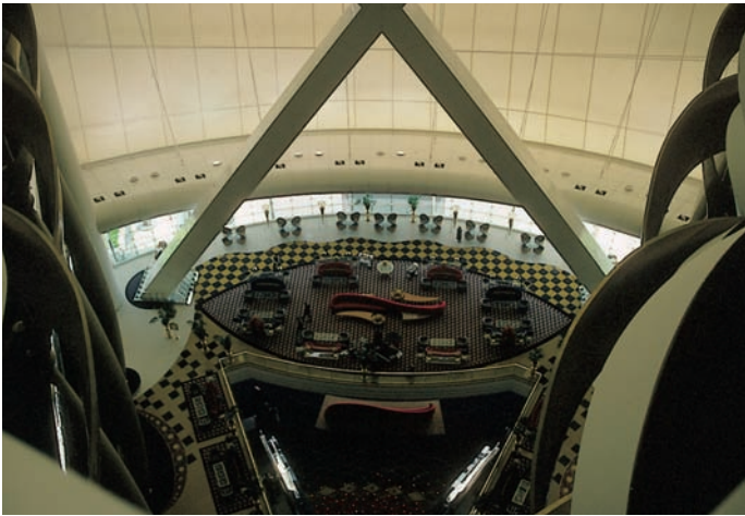
Above Detail showing the conjunction of one of the tower's walls and the atrium's white Teflon screen
