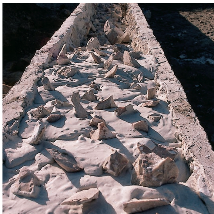
Top Close-up of the imported coral-reef rock used in the reconstruction of Sharjah's vernacular architecture
