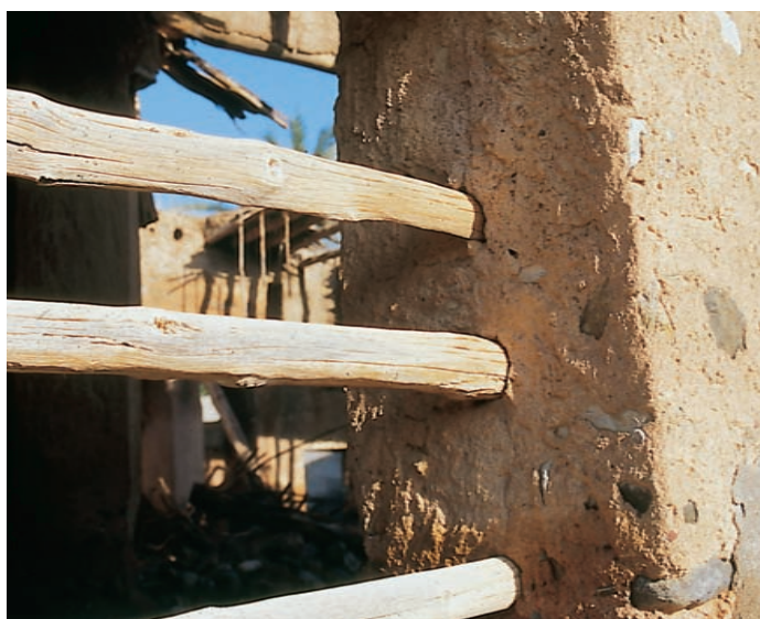
Above Khatt, mosque no. 9: thick branches or tree trunks are used as a grating to stop intruders
