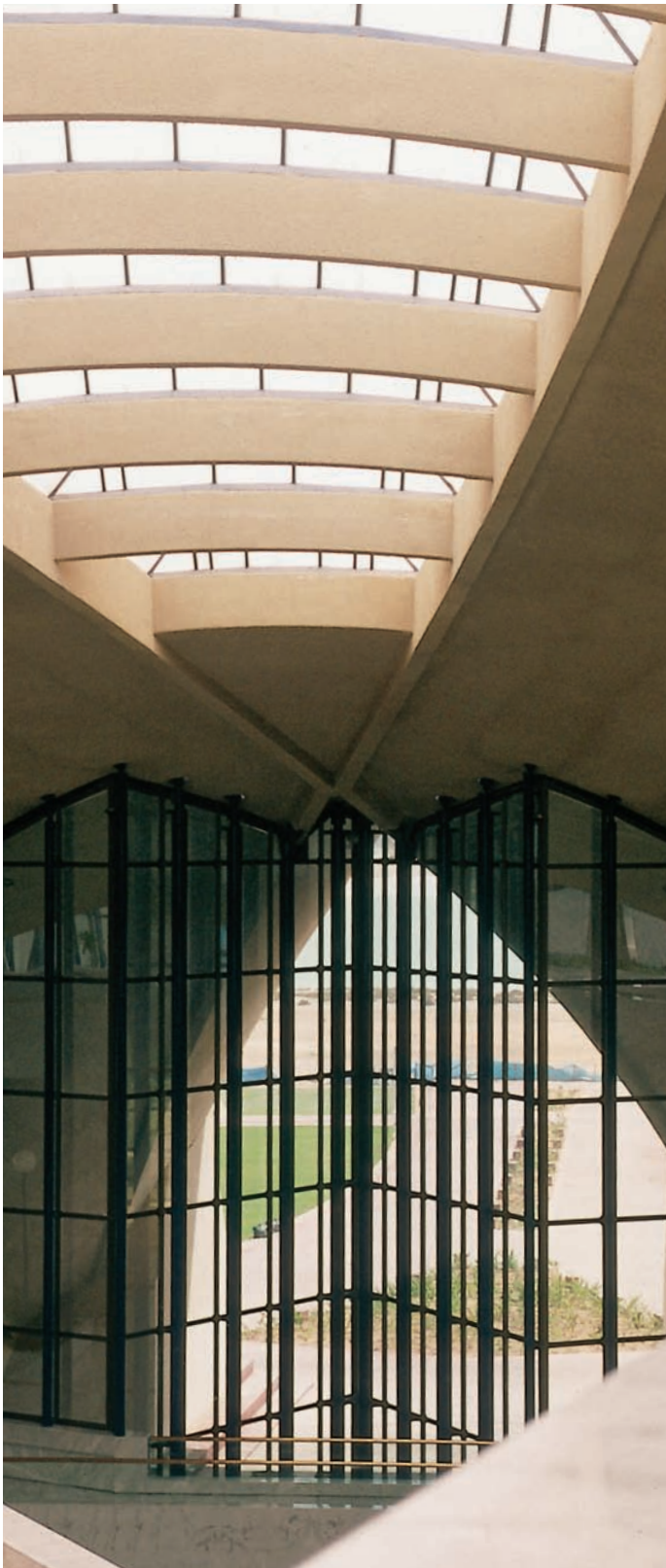
Above Segment of the shell and glass wall joining the structural shell with the skylight above
