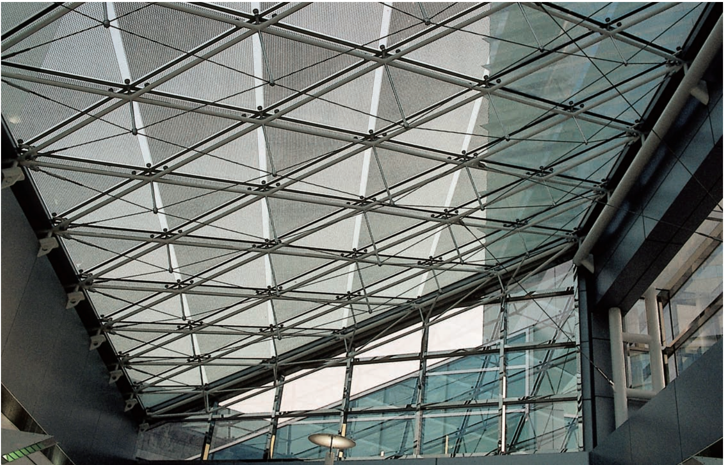
Above Close-up of the glass and steel-frame skylight in the retail mall
