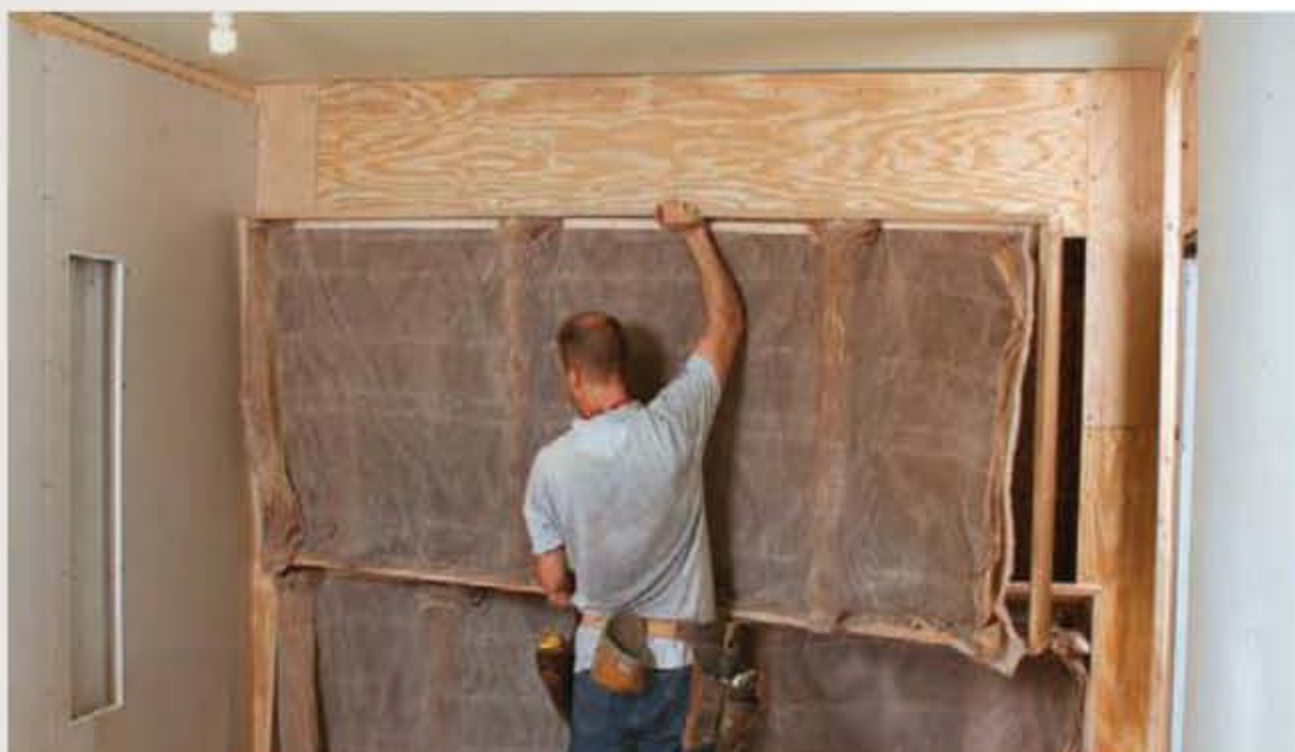
Finally the filters. Filter material (to catch the overspray) is attached to two frames that stack one on top of the other in front of the fan.
