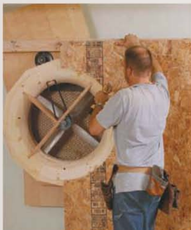
Add the sheathing. Sheets of 1/2-in.-thick OSB form the back of the plenum.
