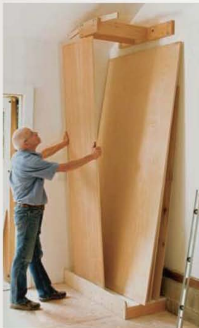
Safe storage for sheet goods. The restraining bars lift out of the way for loading. A lipped platform secures the sheets at the bottom.
