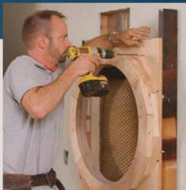
Ring the exit. Attach the mounting plate with the exit ring to the 2x4 studs that surround the exhaust air opening.
