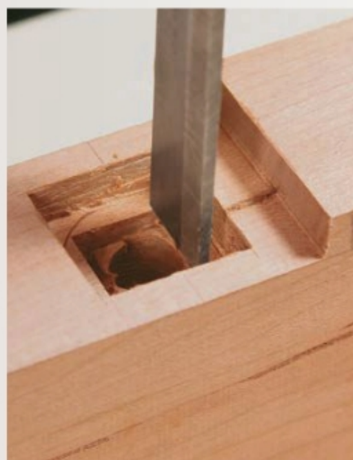
Two holes for a stepped mortise. Drill the larger hole first and then center the smaller bit in the dimple left by the larger one. Use a Forstner bit for both. Square them up, again starting with the bigger mortise before the smaller one.
