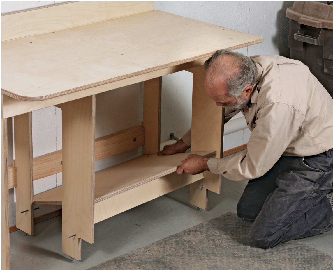
Put the shelf in place. The toe kick and cam locks are already in place. The four dowels should fit into the router slots, supporting the shelf.
