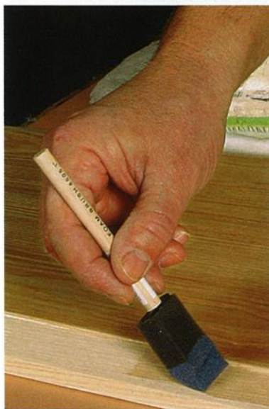
A choice of brushes. When applying a water-based finish to narrow surfaces, use either a foam brush or an artist's brush with man-made bristles.
