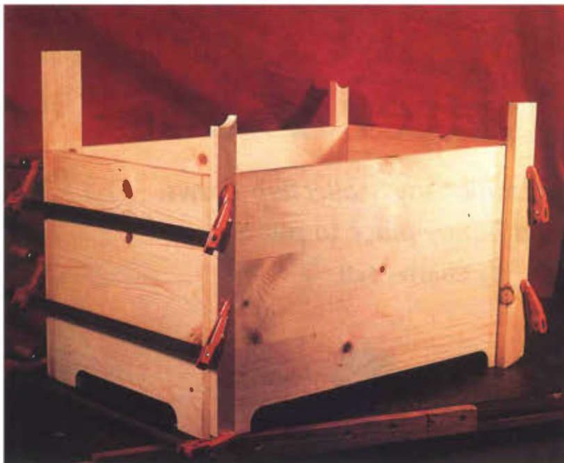
Assemble the box and clamp up until the glue has set.
