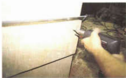
7. The joint board for the corner section may be glued and screwed on, or secured with nails and glue.
