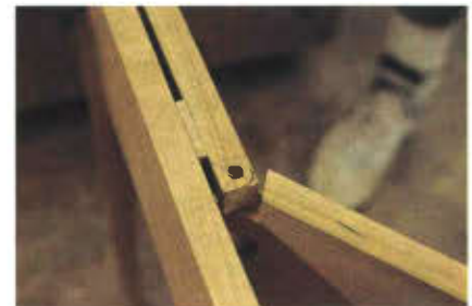
15. Pin in place, this photo shows the working mechanism of the finger-joint gate.
