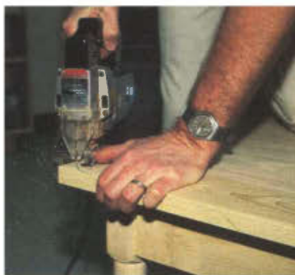
Photo 14. To make the radius cut on the table top corners, first pencil on the finish cut line using the template, then jigsaw cut the waste just wide of the line.
