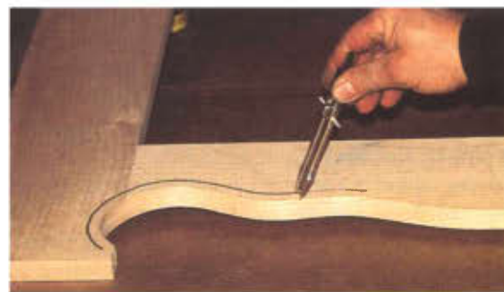
Photo 10. A cockbead can be added prior to hanging the doors by using a compass to mark the line \frac{1}{8} " from the scroll edge, then use a hand grinder or chisel to carve the V-groove.
