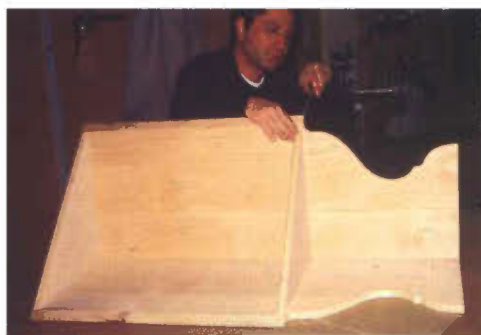
Photo 7. After the back pieces are screwed together, attach the triangular top and bottom using screws or nails from the back of the cabinet.
