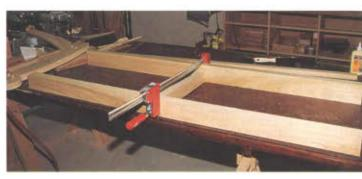
Photo 11 The center seat support is glued and clamped between the front and rear seat stretchers.
