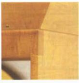
**Photo 1** The assembled dovetail on the top rail joining the case side. The top edge, hidden by the crown, was not dovetailed, but simply nailed to the side.
