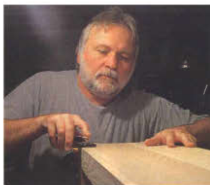
Photo 6 Clamp the face frame in position and hand plane it to an exact fit so that the biscuit joints are cut exactly where they should be cut.
