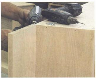
6 SIDE WINGS • Attaching the backs for the side shelves is a little tricky. I used screws angled through the side rabbets. Pilot drill through the rabbet and into the backs or you stand a good chance of splitting out the wood on this angled attachment.
