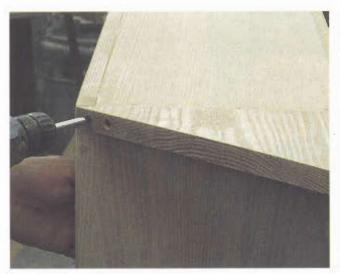
ANGLE TOPS • Install the tops using screws or nails through the front corner of the angled boards. They won't show because the crown moulding will cover that edge. Attach the back edge of the top through the back with screws.
