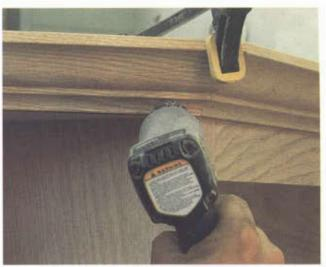
8 THE CROWN • Take your time and make a couple of test cuts on the crown. All that's required is patience to get a nice tight fit. I used a pneumatic nailer to attach the crown quickly and without a lot of clamping.
