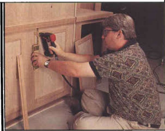
The false doors attach quickly using a brad nailer. Make sure the spacing is even across the face panel.
