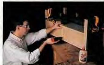
back of the coffee table to look as interesting as the front To mimic the divider on the front of the case, I pinned a piece of moulding in the middle of the back too.
