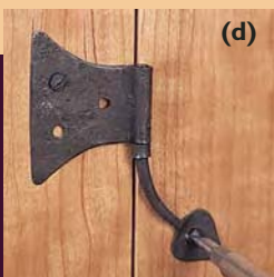
(d). When you've got a good fit, hold the hinge in place and peen the snipe ends over after splaying them with a screwdriver (e).
