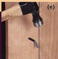
(d). When you've got a good fit, hold the hinge in place and peen the snipe ends over after splaying them with a screwdriver (e).
