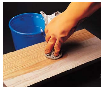
After the board has dried, remove the crystals using a wet rag or a hose. Never brush the crystals off the surface.
