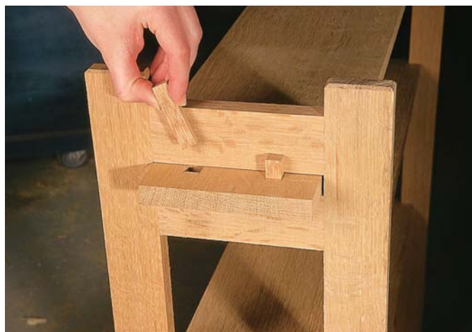
Most of the tapered part of the wedges should slide through each mortise. As the wedge gets wider, you will need a mallet and a block of wood to finish pounding them down to a uniform height.
