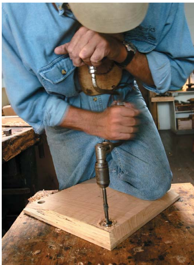
Use your body weight to hold the workpiece in place as you bore the holes for the legs. Beginners should place a square (or two) near the bit to guide their progress.
