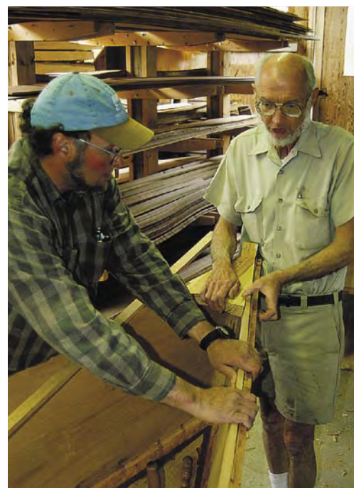
Sarge and I begin the inside work with fitting the small deck block. Together with the inside gunwhale and transom knees, this will contribute stiffness to the hull.
