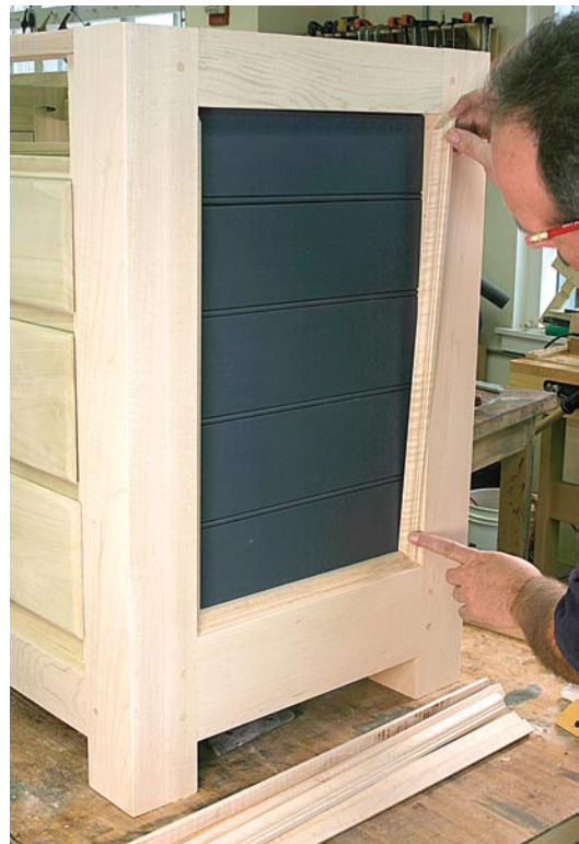
Picture-frame moulding. The panels on the base are held in place by the moulding that is installed in picture-frame fashion – the corners are mitered.
