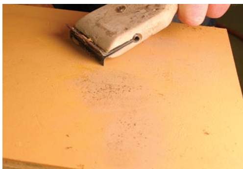
Scrape off the blisters with a common paint scraper. You don't have to use a lot of downward pressure. Stop scraping when you've popped all the blisters off.
