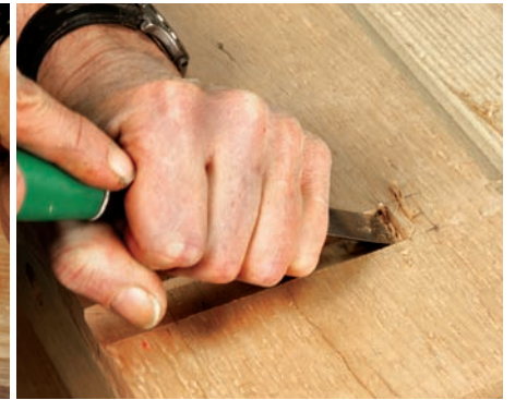
Finish by hand. A few cuts with a chisel complete the end of the dado for the top and bottom shelves. The front edge of the shelf is notched and ends \frac{1}{2} " past the end of the dado. The notch is cut by hand with a dovetail saw.
