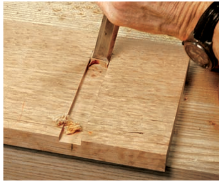
Finish by hand. A few cuts with a chisel complete the end of the dado for the top and bottom shelves. The front edge of the shelf is notched and ends \frac{1}{2} " past the end of the dado. The notch is cut by hand with a dovetail saw.
