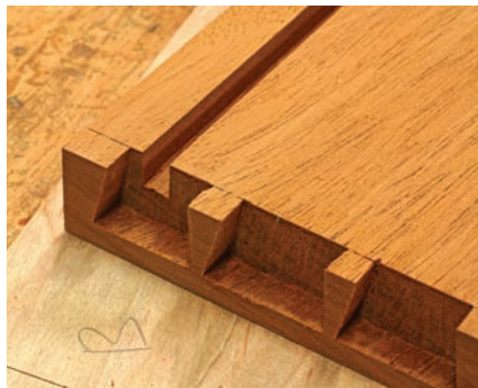
In the groove. The slot for the drawer bottom is located in the space for the lowest tail in the drawer front.
