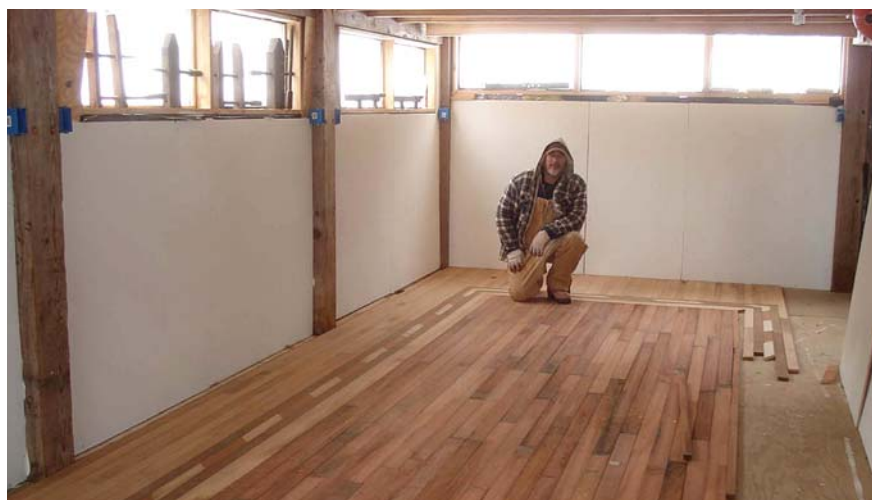
Fancy. The palace parquet won't look out of place, because the rest of the barn's flooring is fancy, too. Here, I'm installing madrone flooring with an oak surround (all salvaged stock, of course).
