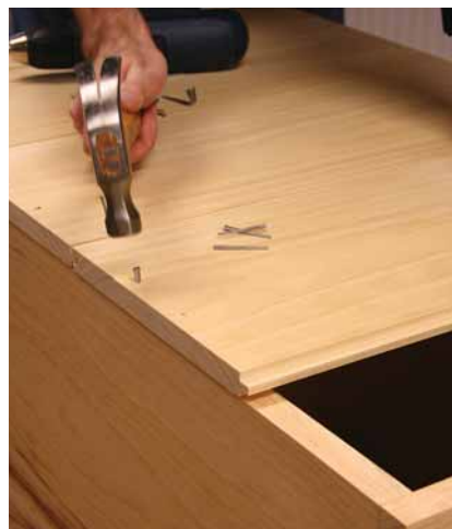
Fixable. By securing the bottom with nails instead of a fancier joint, you are making the chest easier to repair in the future. Bottom boards can rot.
