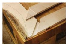
**Super-strong joints.** Although it's a break with tradition, mitered half-lap joints add support to the base-frame mouldings and simplify how the return mouldings are attached.
