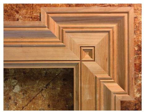
**Hip to be square.** A detail shows how the four parts of the crossette form a makeshift rosette at each corner. Although no finish has been applied here, the chatoyant differences of light reflected from the surfaces are already visible.
